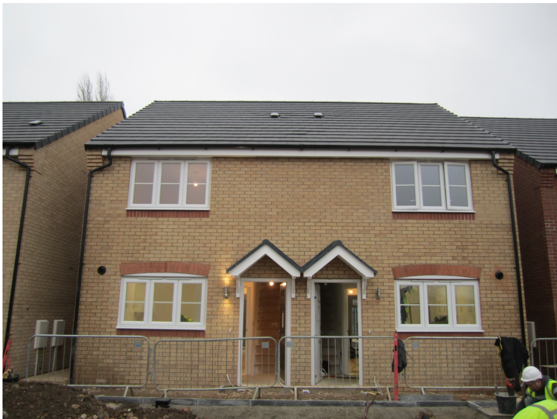
New Council homes under construction at Vincent Court.
